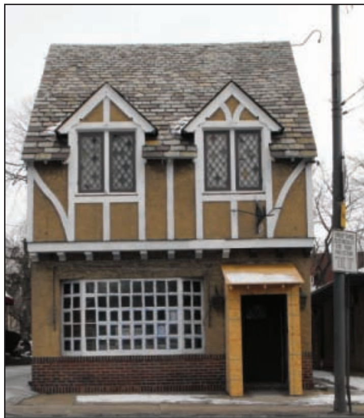
Before (left) and in-progress improvements at 47 S. Lansdowne Avenue
