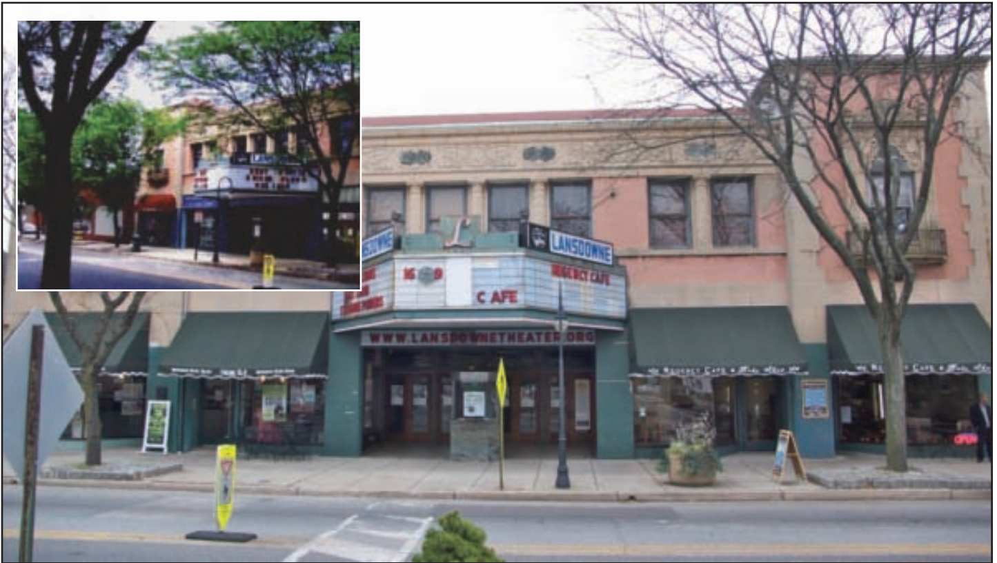
The Lansdowne Theater before (inset) and after improvements.
