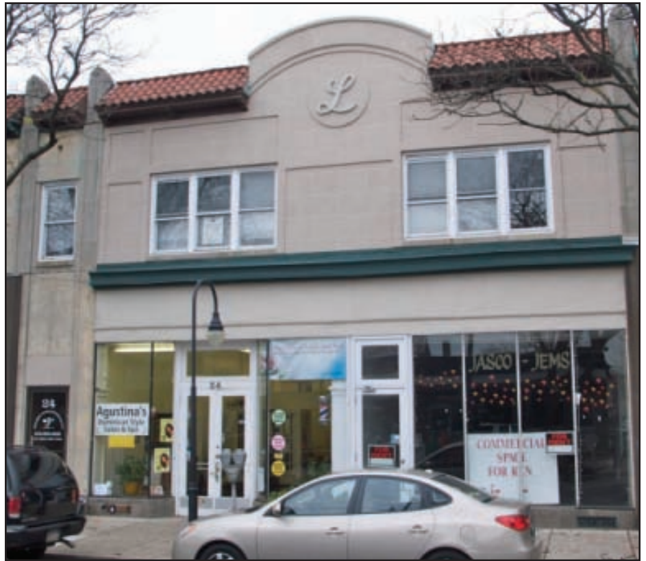
Before (left) and after improvements to storefronts at 24-26 N. Lansdowne Avenue
