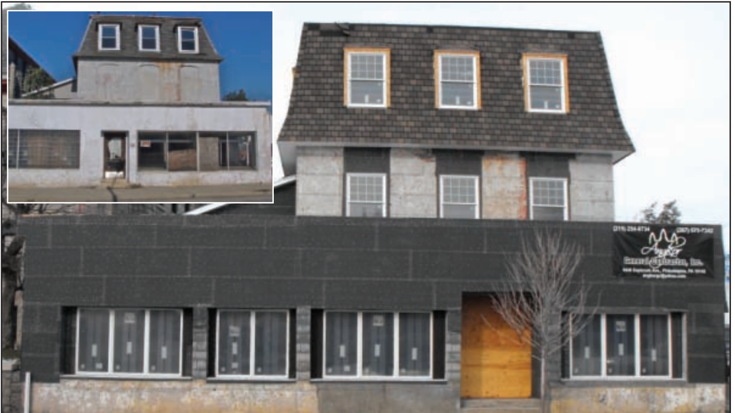
Before (inset) and in-progress improvements at 55 E. Baltimore Avenue
