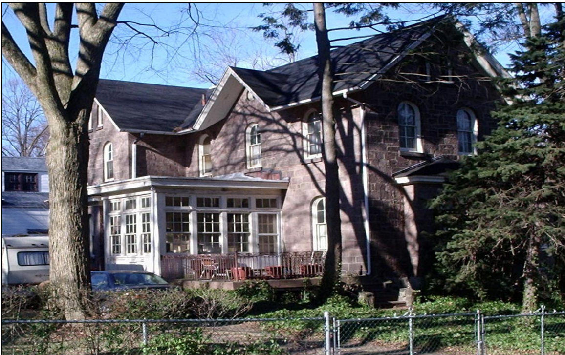
Willowbrook in Lansdowne, an example of early mansion development
