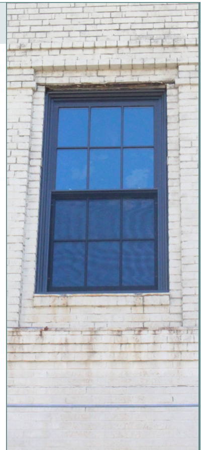
The six-over-six new windows above were used to replace the originals, pictured below, at 32 E. Baltimore Ave.
